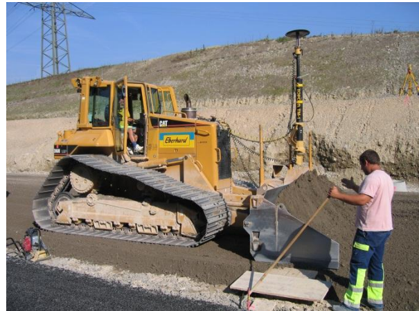
Figure 5.2 Dozer with prism for height control with tachymeter. Picture (D. Grimm)
