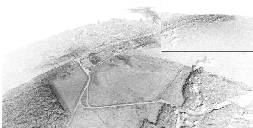
Fig. 7 Reconstructed dense point cloud based on the combination of the oblique-view grayscale camera images with the vehicle position estimates. The reconstruction was achieved using the Pix4D mapping software.
