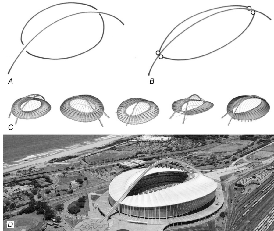
Figure 3.14: Moses Mabhida Stadium. (A) Initial structural concept, (B) final structural concept, (C) intermediate states of the analysis model during the design process (Balz, Göppert et al. , 2009: 1232, 1233), and (D) photo of the realised project (Bögle, Breising et al. , 2011: 23).
