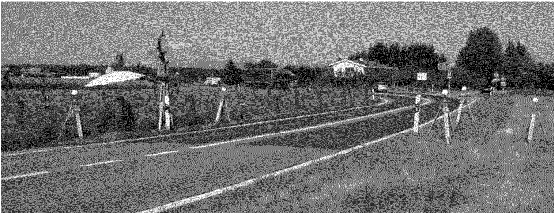
Figure 6.1: Road section to be investigated. Control points, visualized by spheres and mounted on tripods, can be seen.
