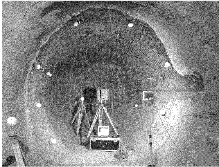
Figure 6.7: Laser scanner inside the excavated niche including object points signaled by spheres.
