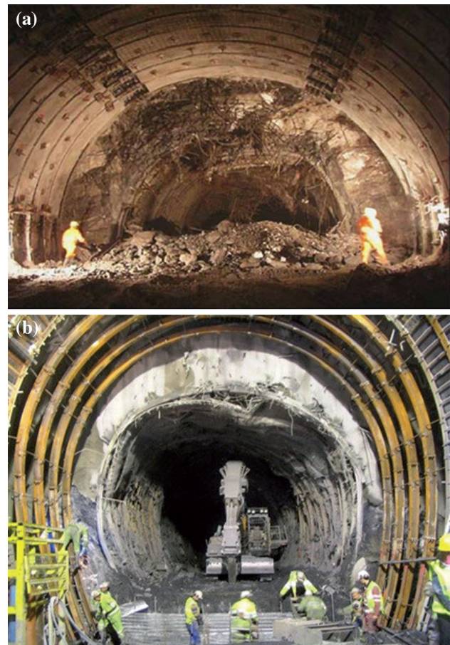
Fig. 1 Examples of tunnels necessitating re-profiling: a multifunctional Faïdo station, Gotthard base tunnel, Switzerland (Ehrbar 2008); b Saint Martin La Porte access adit, Lyon–Turin base tunnel (Rettighieri et al. 2008)
