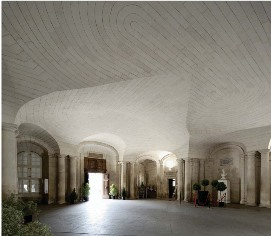
Figure 2.27: The complex, discrete stone vault of the City Hall in Arles, France, 1676, by Jules Hardouin-Mansart. (Image: Brandon Clifford, 2011)
