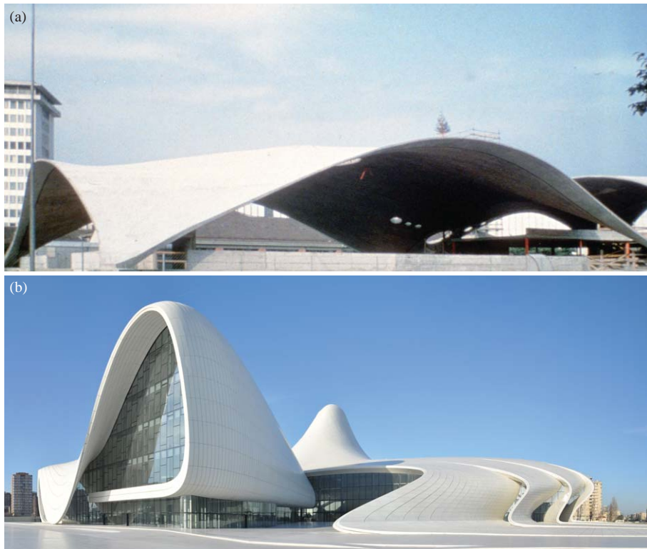
Figure 2.5: Funicular and freeform architecture: (a) The Sicli company building under construction, Geneva, Switzerland, by Heinz Isler (1969), (b) Heydar Aliyev Center, Baku, Azerbaijan, by Zaha Hadid Architects (2012). (Images: (a) Heinz Isler, (b) Markus Wilthaner)
