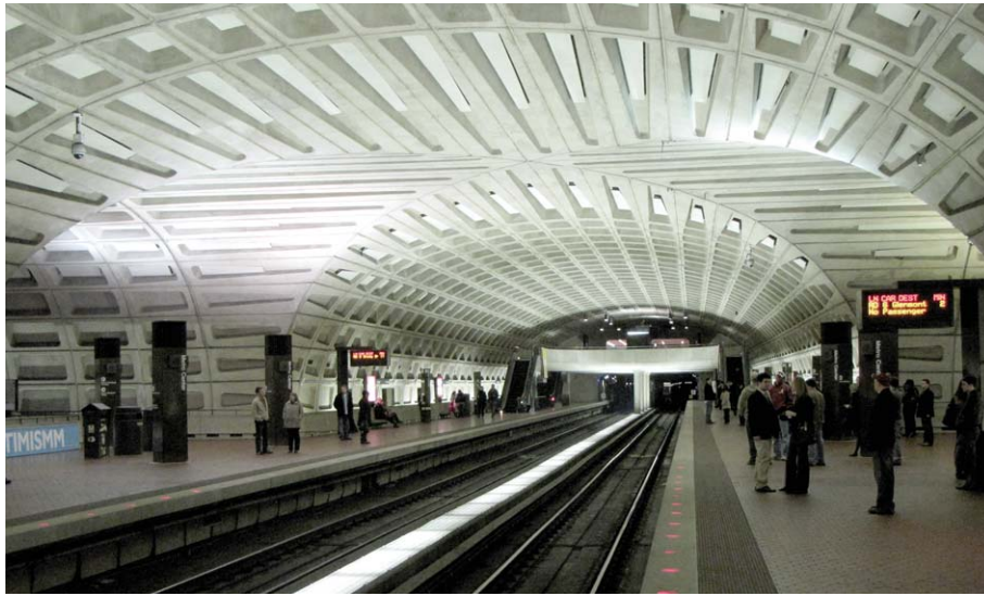
Figure 2.31: Intersection of coffered concrete ceiling vaults at Metro Center Washington, D.C., USA (1976) designed by Harry Weese (Image: Ben Schumin).
