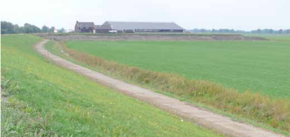
Recently built "terp" at the southern edge of the Overdiepse Polder (Rossano, 2013)
