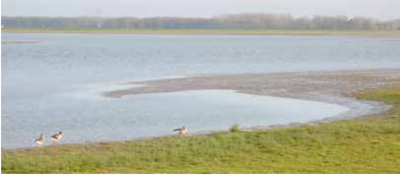
New water inlet in the former Noordwaard polder (photo Rossano, 2012)
