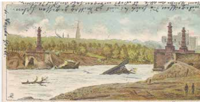
Munich, collapse of the Prinz-Regenten Bridge during the 1899 high waters. Postcard, detail, 1899 (collection of the author)
