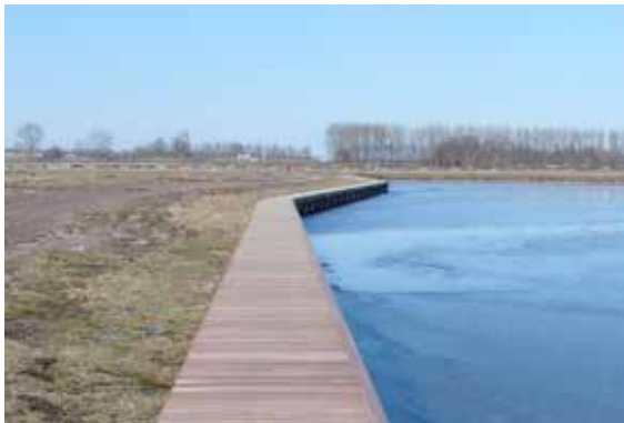
Meerstad: promenade between building land and new recreation/mitigation lake (Rossano, 2013)
