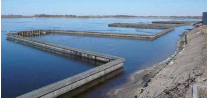
Meerstad, island under construction (Rossano, 2013)
