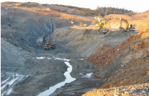
Fig 5. Excavation of the Kearney Vein. (Galantas, 2014)
