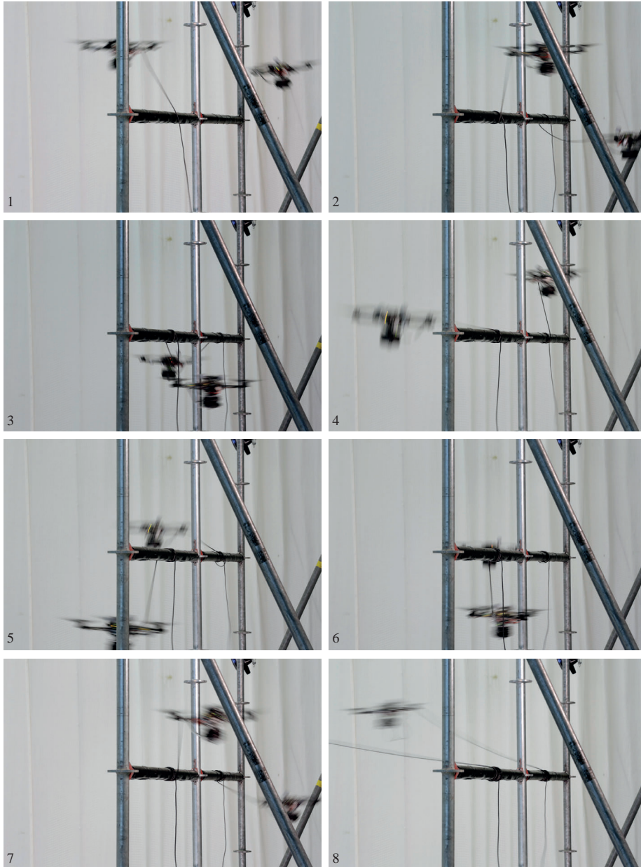
Fig. 5.19: Parallel knot construction of the first knot of the handrail links to the support scaffolding [144].
