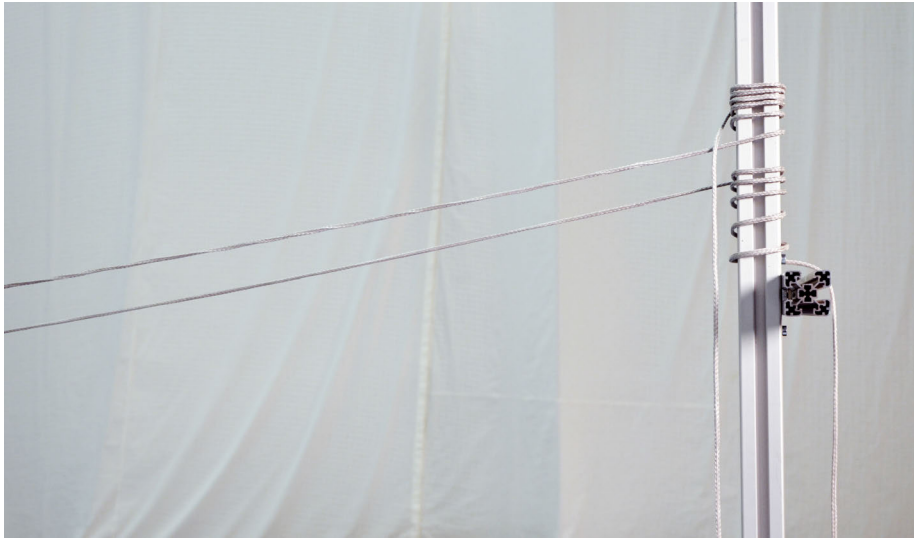
Fig. 5.6: Detail of the constructed knots on a vertical support profile.
