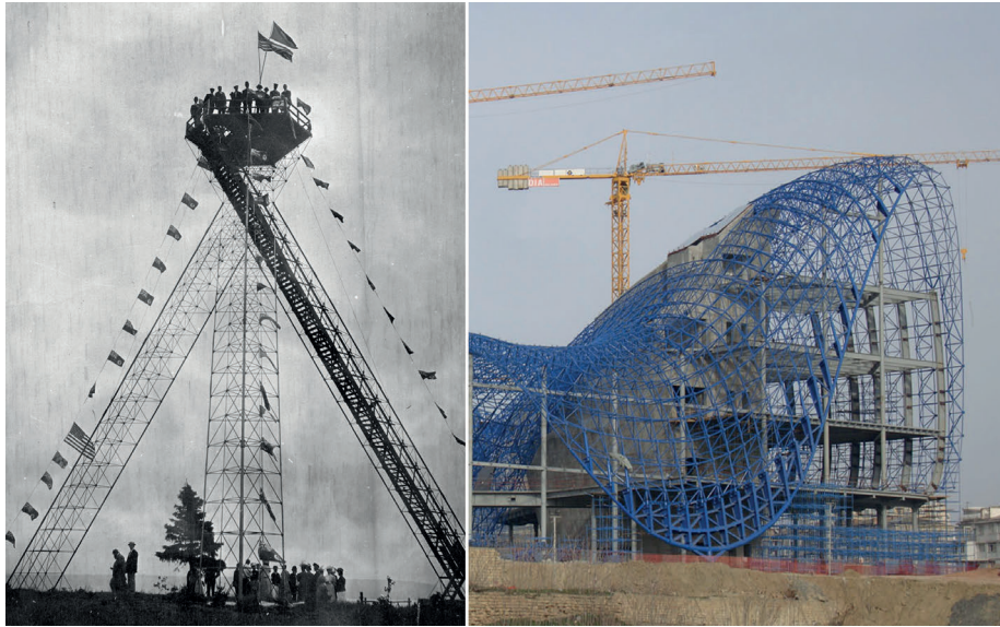
Fig. 3.5: Tetrahedral tower by Alexander Graham Bell unveiled in 1907 in Cape Breton Island, Nova Scotia, Canada. Free-form MERO [90] construction system at the Heydar Aliyev Centre in Baku, Azerbaijan by Zaha Hadid Architects, during construction in 2011 [91].
