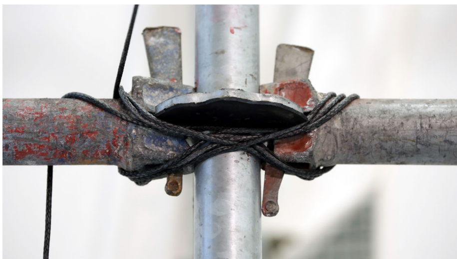
Fig. 5.22: Constructed starting knot of the footrope link. A series of diagonal turns cross the centre point of the knot.
