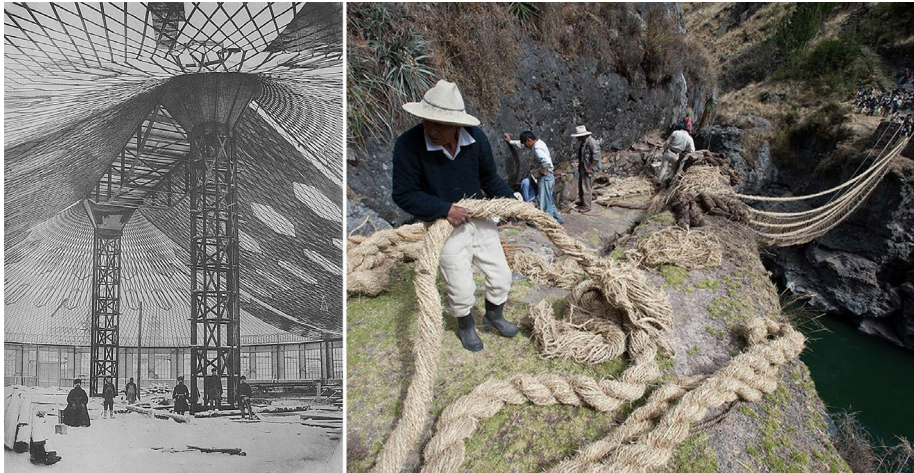
Fig. 3.6: On the left, a view of the Tensile Steel Diagrid Shell of the Oval Pavilion by Vladimir Shukhov during construction in 1895. On the right, a villager constructs a new bridge over the Apurimac River in Huinchiri (Peru) in 2012.
