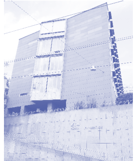
IFW: the new ETH building
