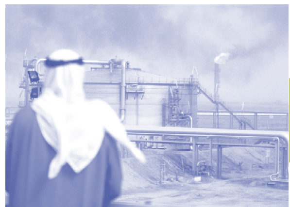
Oil-plant in Saudi Arabia. (Photo courtesy of INEWP)
