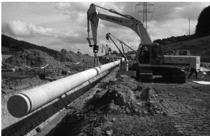
Fig. 5.1. Placement of sections of pipeline.
