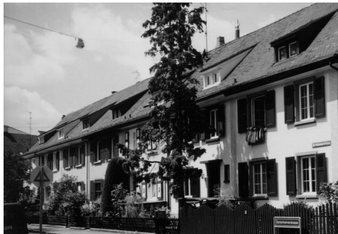
Figure 6.14: Real example building from the city of Basel
