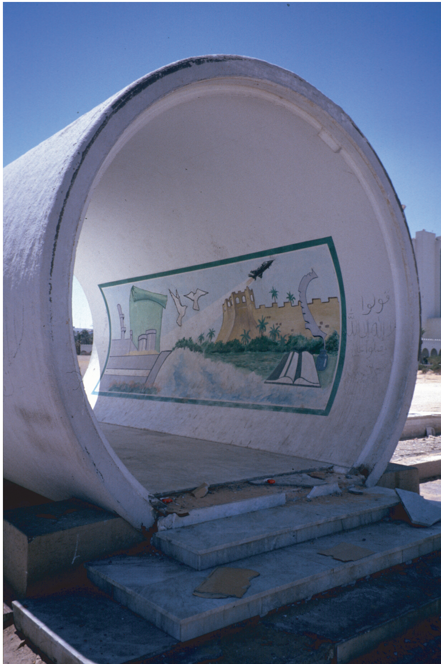
Figure 4.1: Conveyance pipe segment of the Great Man Made River-Project as displayed in Tripoli. The concrete pipes are pre-stressed steel wire enforced. The artwork inside the pipe segment depicts the successful struggle of the Libyan people against foreign aggressors while enjoying the benefits that result from the greening of the desert.
