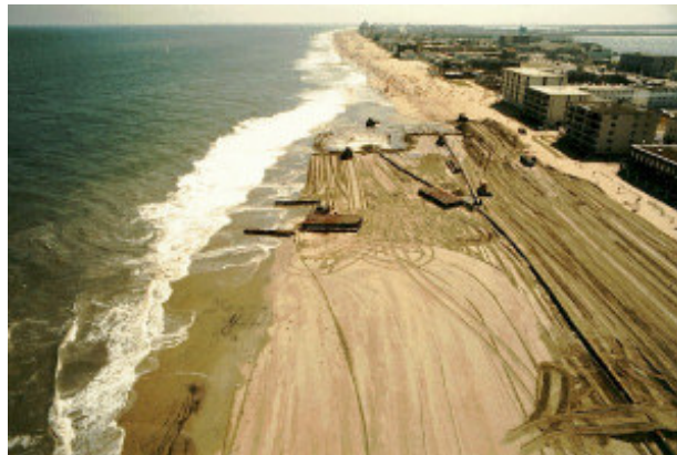
Figure 5.16: Example of a protection option: beach nourishment in Ocean City, USA (Rutgers Institute of Marine & Coastal Sciences, 2001).
