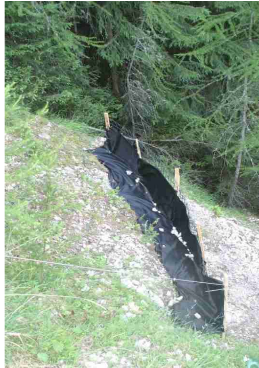
Figure 4-7 Silt fence plot A1 (Corina Gwerder)
