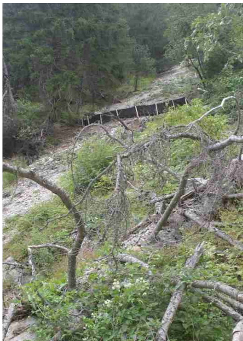
Figure 4-20 Silt fence plot E1 (Corina Gwerder).
