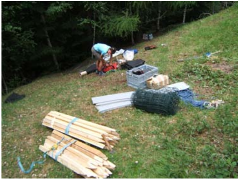
Figure 4-27 Installation work 1, (Corina Gwerder)
