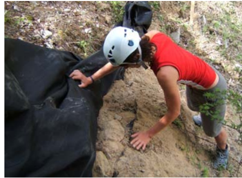
Figure 4-28 Installation work 2 (Corina Gwerder)
