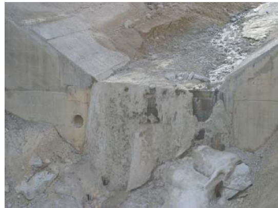
Figure 3-5 The force plate at the Kantonsstrassenbrücke (frontal perspective) (Corina Gwerder)
