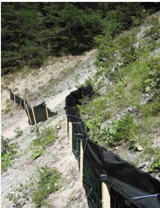
Figure 4-2 Silt fences F1 and G1 (Corina Gwerder)
