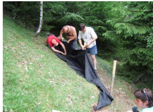
Figure 4-32 Installation work 6 (Corina Gwerder)
