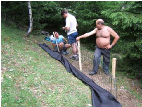
Figure 4-31 Installation work 5 (Corina Gwerder)
