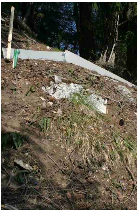
Figure 4-14 Silt fence plot C2 (Corina Gwerder).
