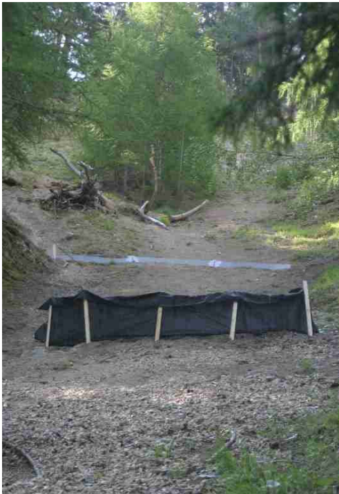
Figure 4-18 Silt fence plot D2 (Corina Gwerder)
