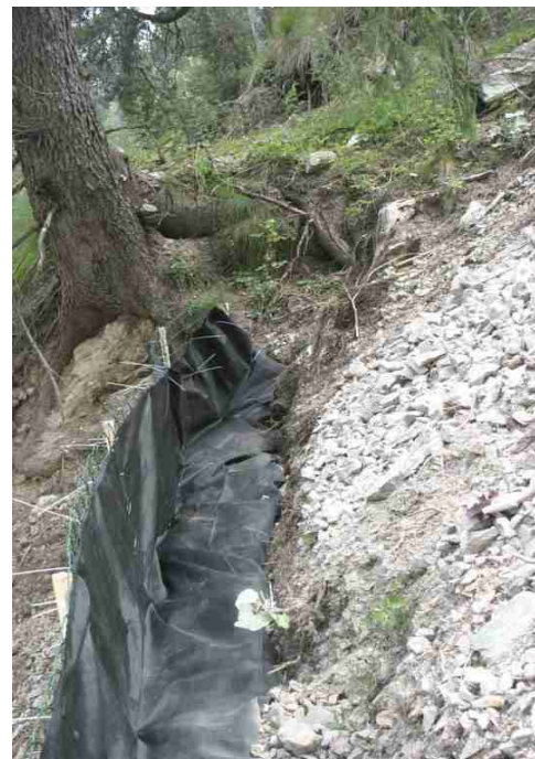
Figure 4-21 Silt fence plot E1 (Corina Gwerder)
