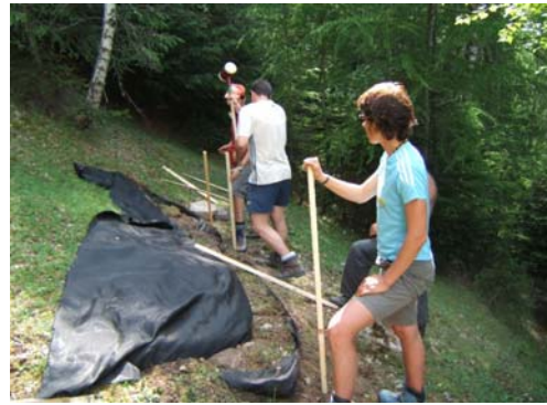
Figure 4-30 Installation work 4 (Corina Gwerder)
