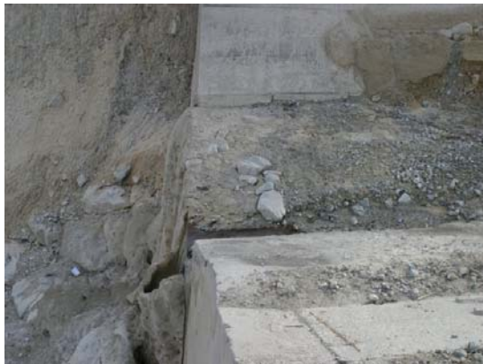
Figure 3-4 The force plate at the Kantonsstrassenbrücke (Corina Gwerder)
