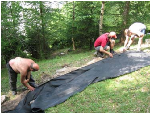
Figure 4-29 Installation work 3 (Corina Gwerder)
