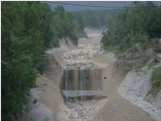
Figure 2-6 Debris flow event 28.07.06 at the Illgraben: the front approaching check dam (Corina Gwerder)
