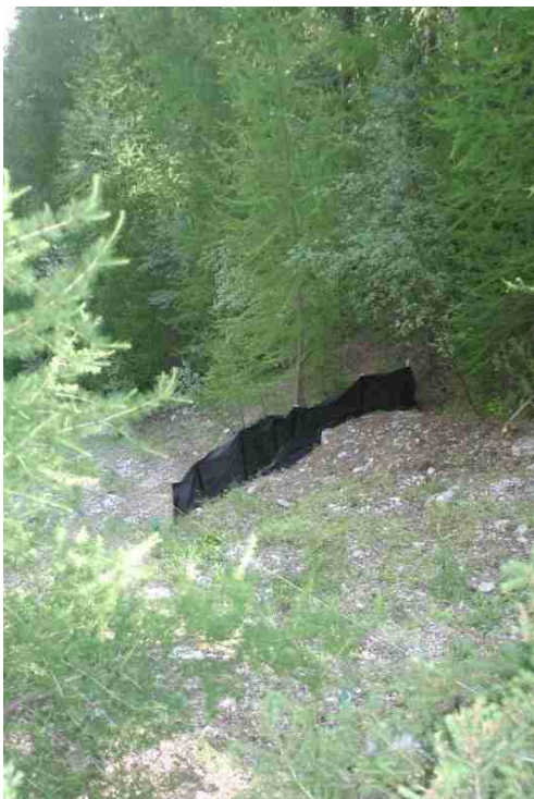
Figure 4-8 Silt fence plot A2 (Corina Gwerder).
