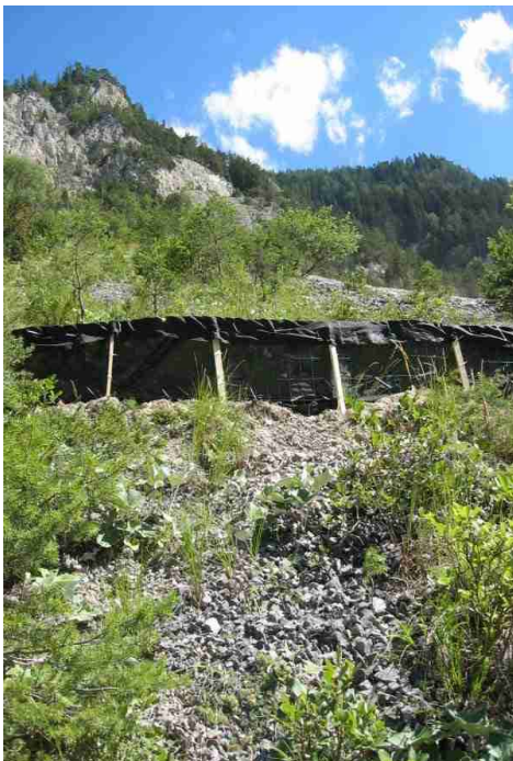
Figure 4-22 Silt fence plot F1, view from below (Corina Gwerder)
