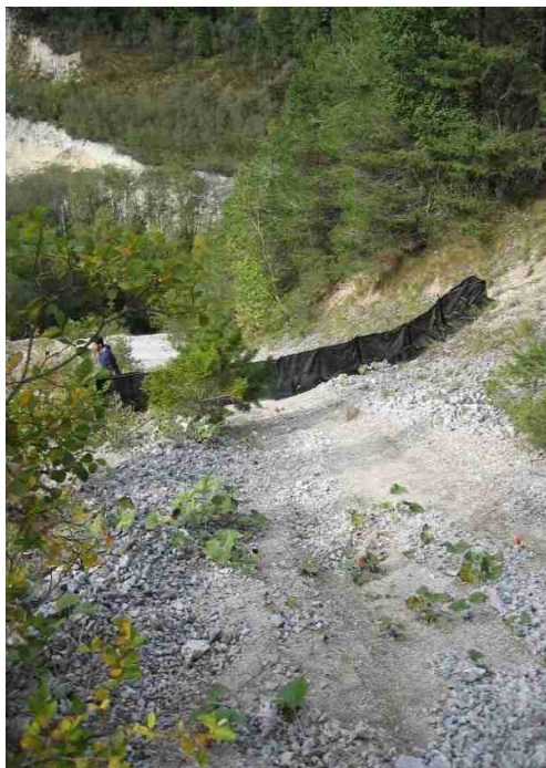
Figure 4-24 Silt fence plot G1 (Corina Gwerder)
