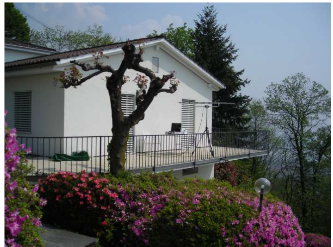
Fig. 1. Horizontally mounted logarithmic periodic dipole on a tripod at the terrace of IRSOL building in Locarno Monti.
