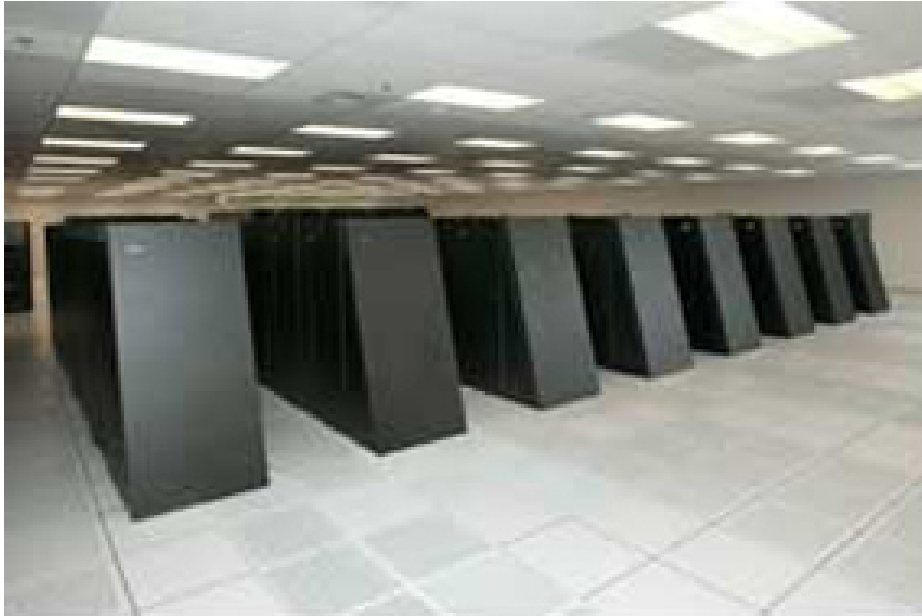
Figure 1.1: Blue Gene/L is housed at the Terascale Simulation Facility (TSF) at Lawrence Livermore National Laboratory: Two supercomputers occupy an entire floor of the 23,504m 2 building (Blue Gene/L machine floor space is 232m 2 ), a second floor is devoted to the housing of cooling devices: “A total of 28 air-handling units blow cool air up to the second level, each at a rate of 80,000 cubic feet per minute”. Adapted from http://www.llnl.gov/asc/asc_index.html
