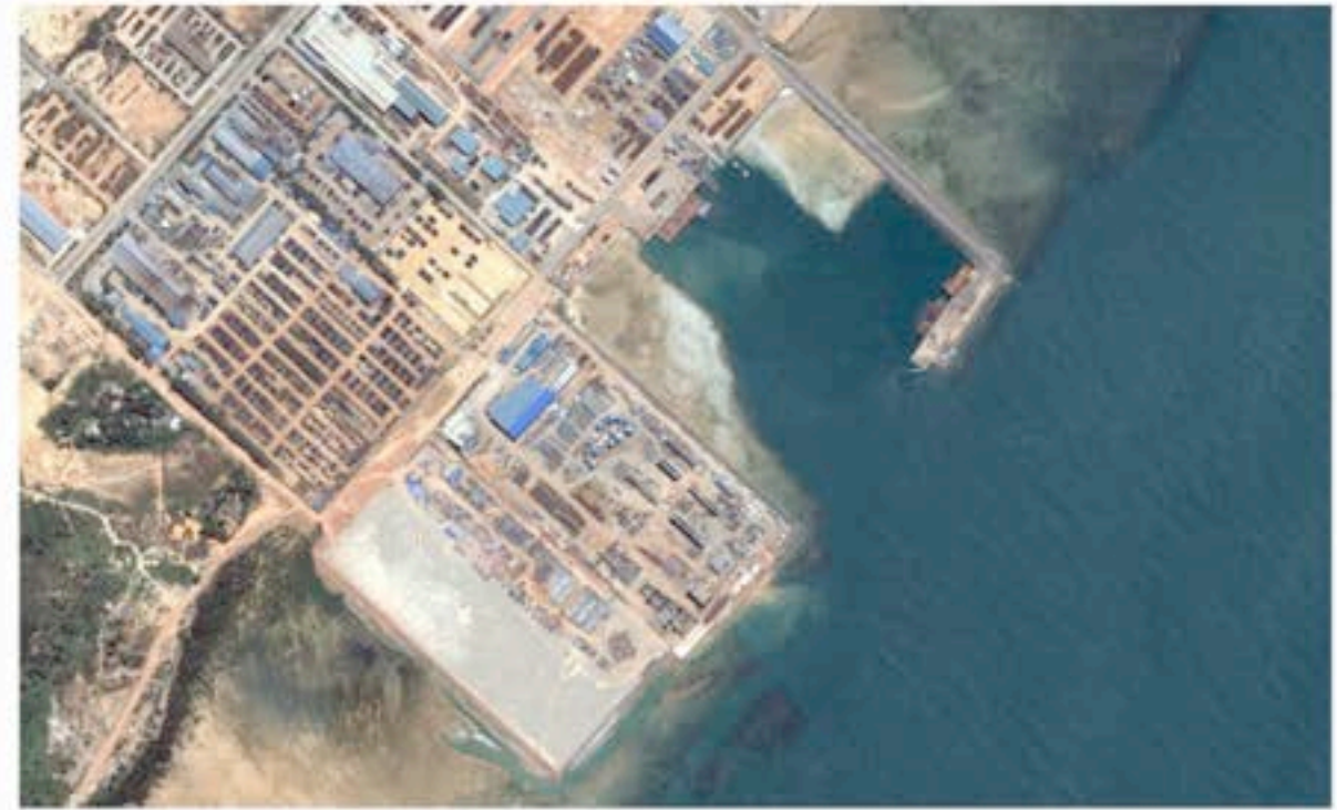
Kabil Industrial Estate Google satellite image
