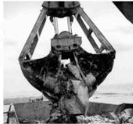
Large clay lumps are taken from the seabed and dumped into construction sites by bottom opening barges.
