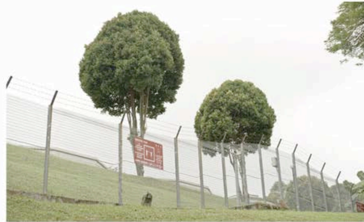
Left: Restricted service reservoir in Fort Canning Park
