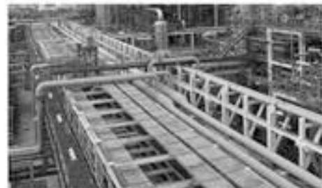
Left: Semboorp Pipeline
