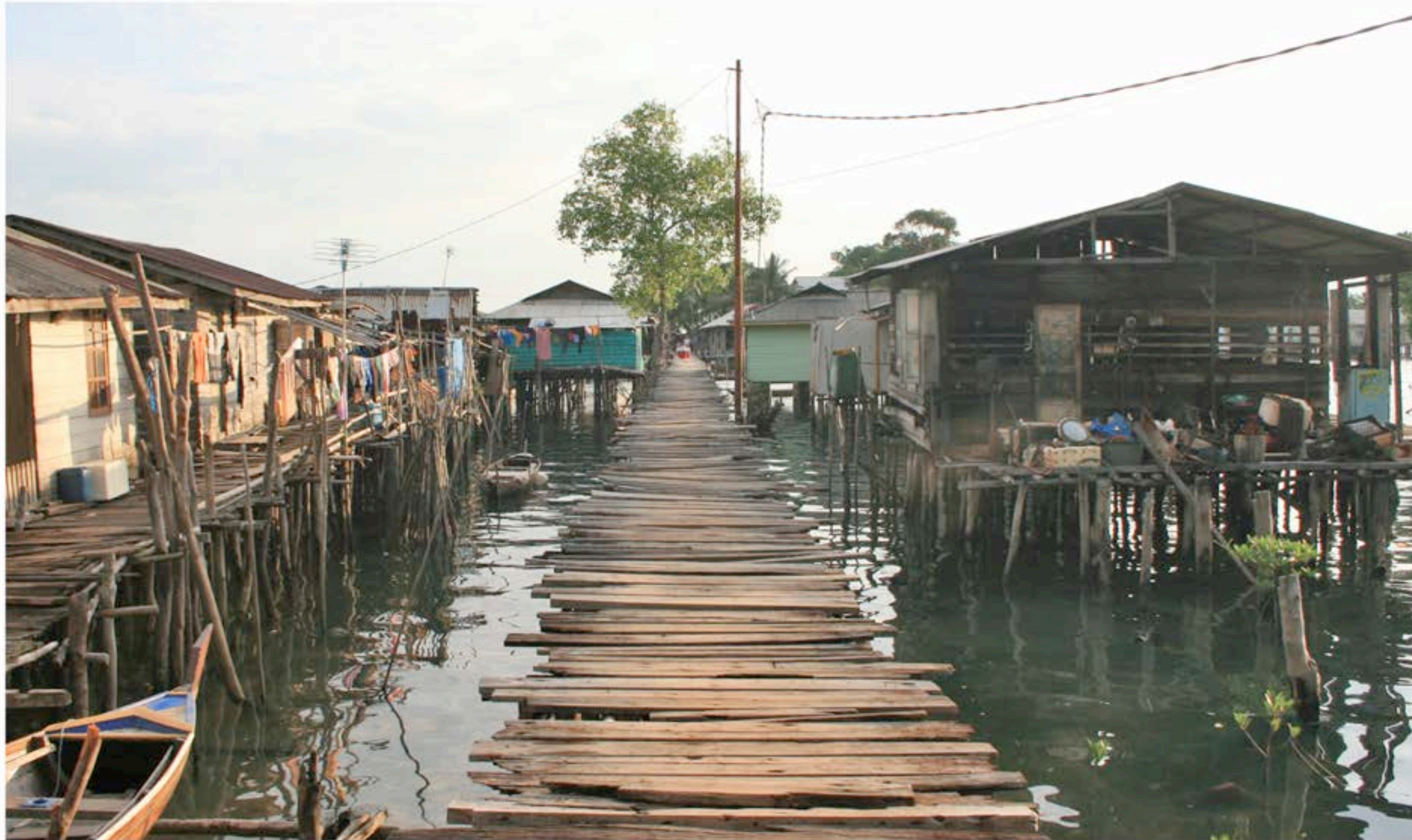
Footbridge, 2012 Kasu Island
