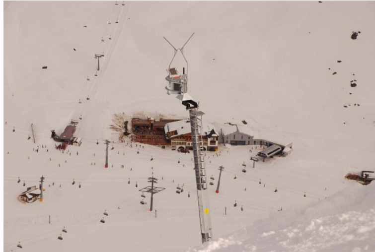
Fig. 1-1: Typical situation where artificial avalanche release (here a fixed system) is used to protect humans and infrastructure.
