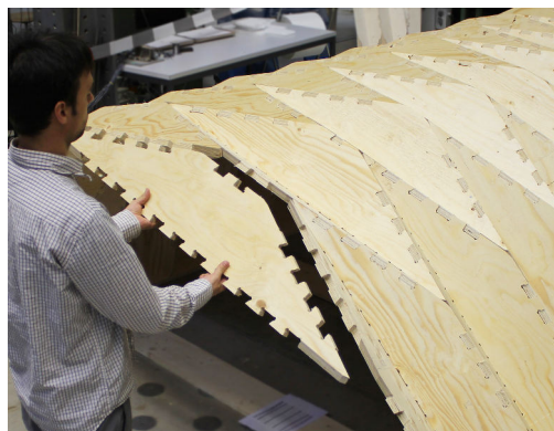
Figure 3: Timber folded plate built from 21mm LVL panels, assembled manually, IBOIS, EPFL, 2014
