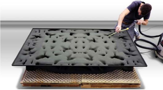
Figure 11. Post-processing of the 3D-printed formwork.
