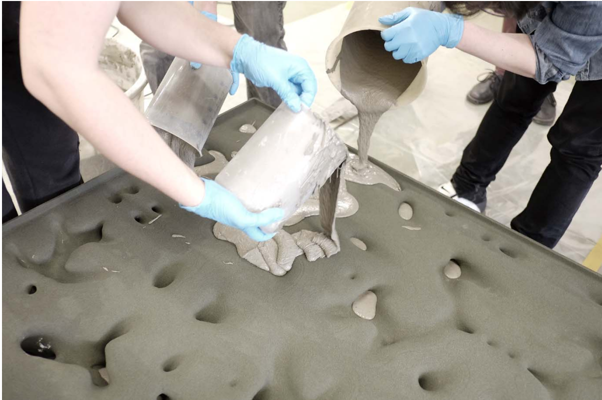
Figure 2. Casting of ultra-high-performance fibre-reinforced concrete in 3D printed sandstone formwork.
