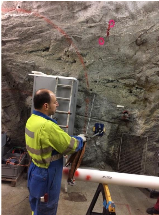
Figure B-5: Installation using winch and pulley
