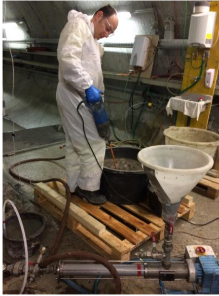
Figure B-10: Grout mixing
