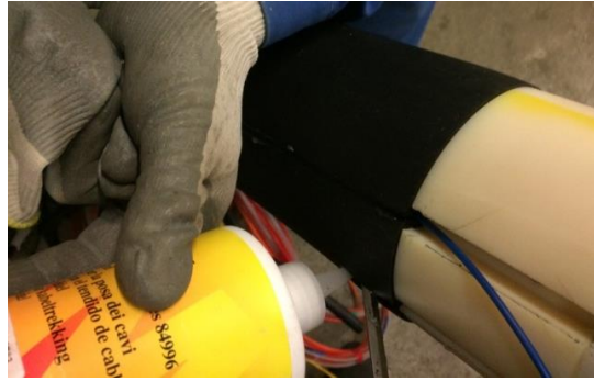
Figure B-4: Fibre optic strain cable passed through packer sleeve
