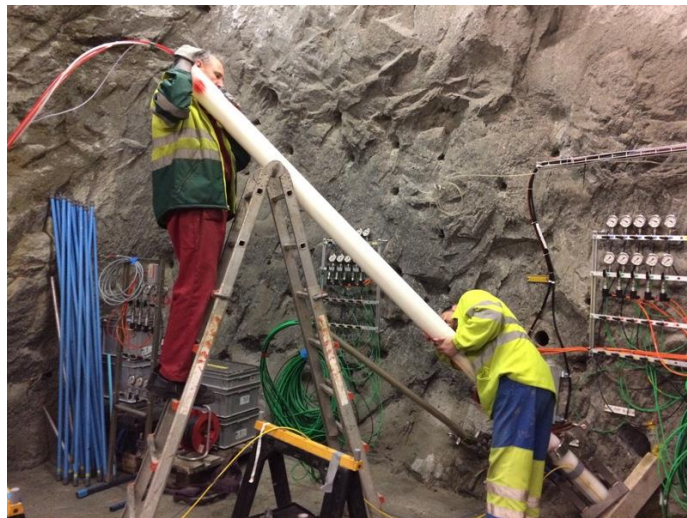
Figure B-12: Installing 2 meter long tube of PRP 16.001 system
