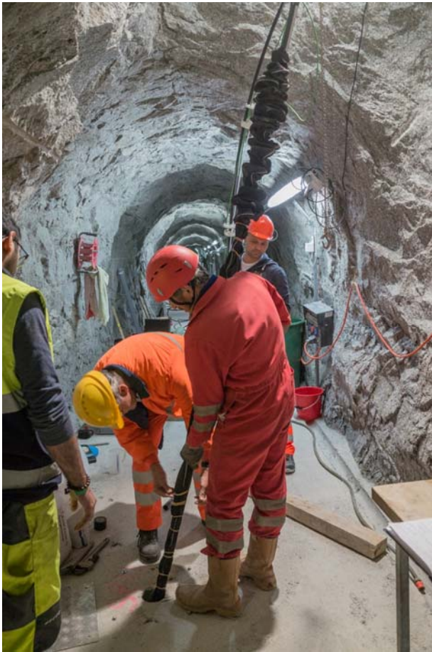
Fig. 7. Compacting the geotextile sleeve with rubber bands to reduce friction.
