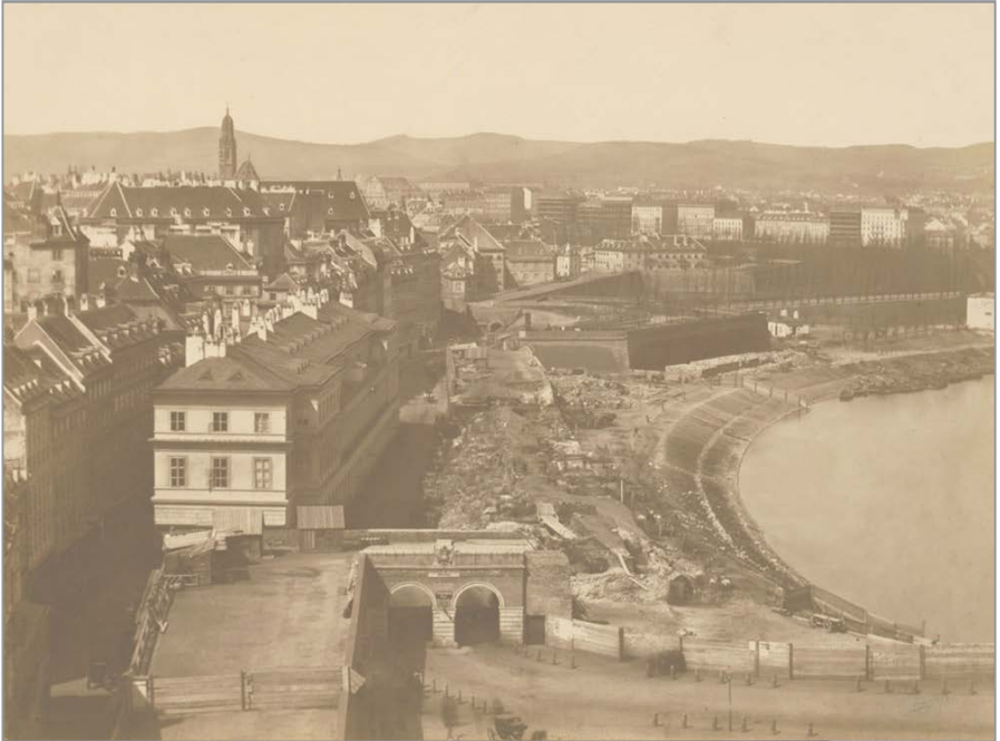
Fig. 2-3 Imperial State Printing Office, Rothenthurmbastei before demolition, 1858, and during demolition, April 1858 (Vienna, Wien Museum)
