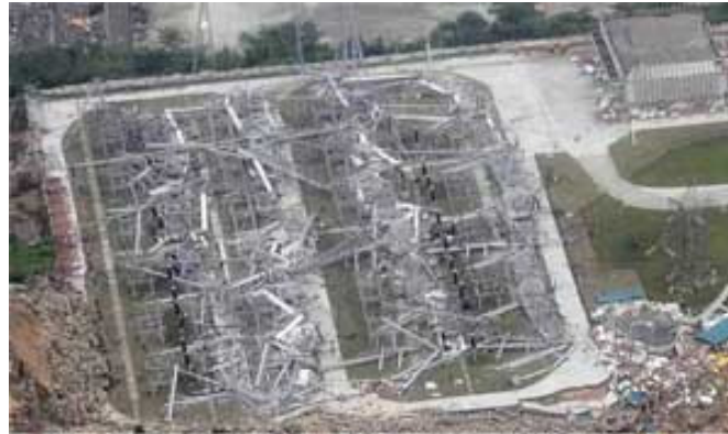
Fig. 2.2. Damaged power substation during Wenchuan Earthquake 2008 (Xie and Zhu 2011)
