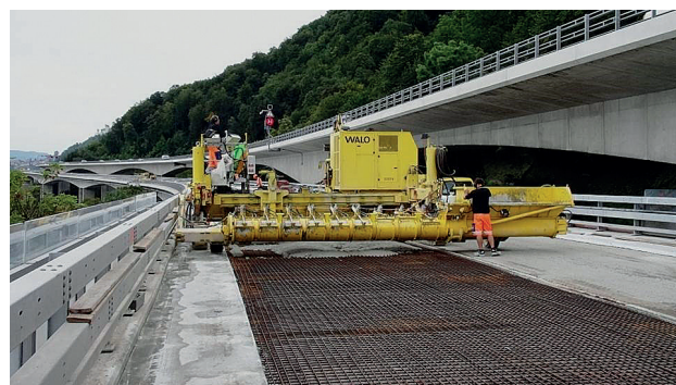
UHFB Rehabilitation Projekt (Chillon Viadukt). UHPFRC Rehabilitation Project (Chillon Viaduct).
