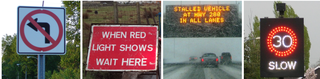
FIGURE 2.1: Examples of existing road sign infrastructure. From left to right: traditional static sign, temporary static sign, variable-message sign, vehicle activated sign. All images courtesy of www.wikipedia.org
