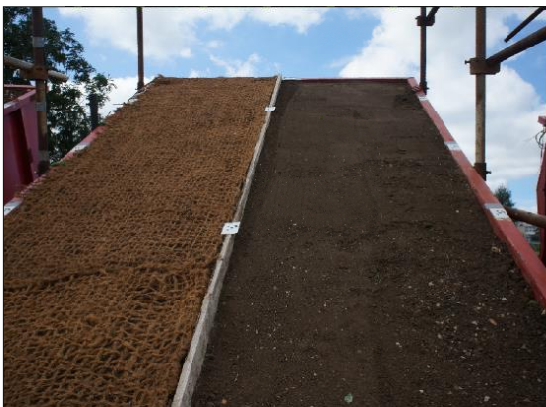
Fig 1: Experimental setup for evaluation of the effectivity of the protection surface cover. On the left is the surface protected with jute geotextile, on the right bare unprotected slope.
