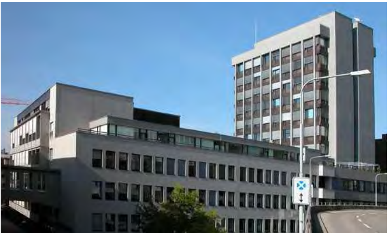
Building CHN on Universitätsstrasse housing the Department for Environmental Science. The IAC occupies the top five floors of the tower building. On the rooftop there is a meteorological station and a balloon launch facility.
