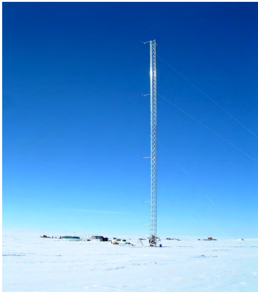
Research tower by the Institute for Climate Research on Greenland Summit, the tallest meteorological tower ever constructed on a glacier
