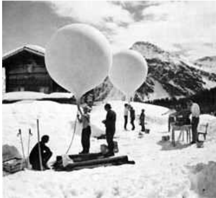
Intercomparison at Arosa of radiosondes with ozone sensors.
