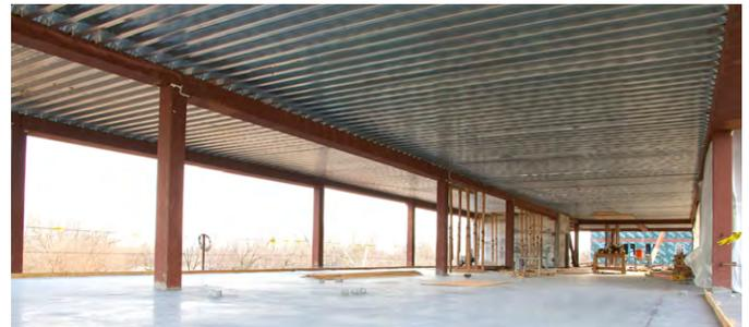
Figure 1: An example long span composite floor system used in modern buildings (Versa-floor, developed by New Millennium Building Systems, LLC) [6].
