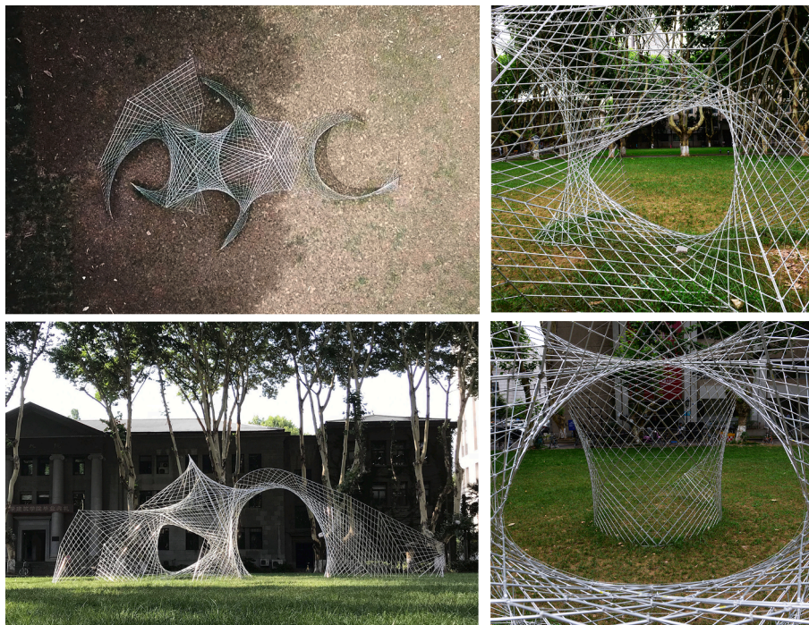
Fig. 16. Pictures of the assembled Hypar Pavilion at the Southeast University of Nanjing (China).
