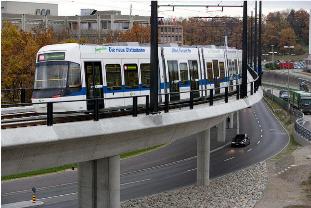
Picture 3 ROW Category A: fully separated way (Glattalbahn viaduct, Zurich)
