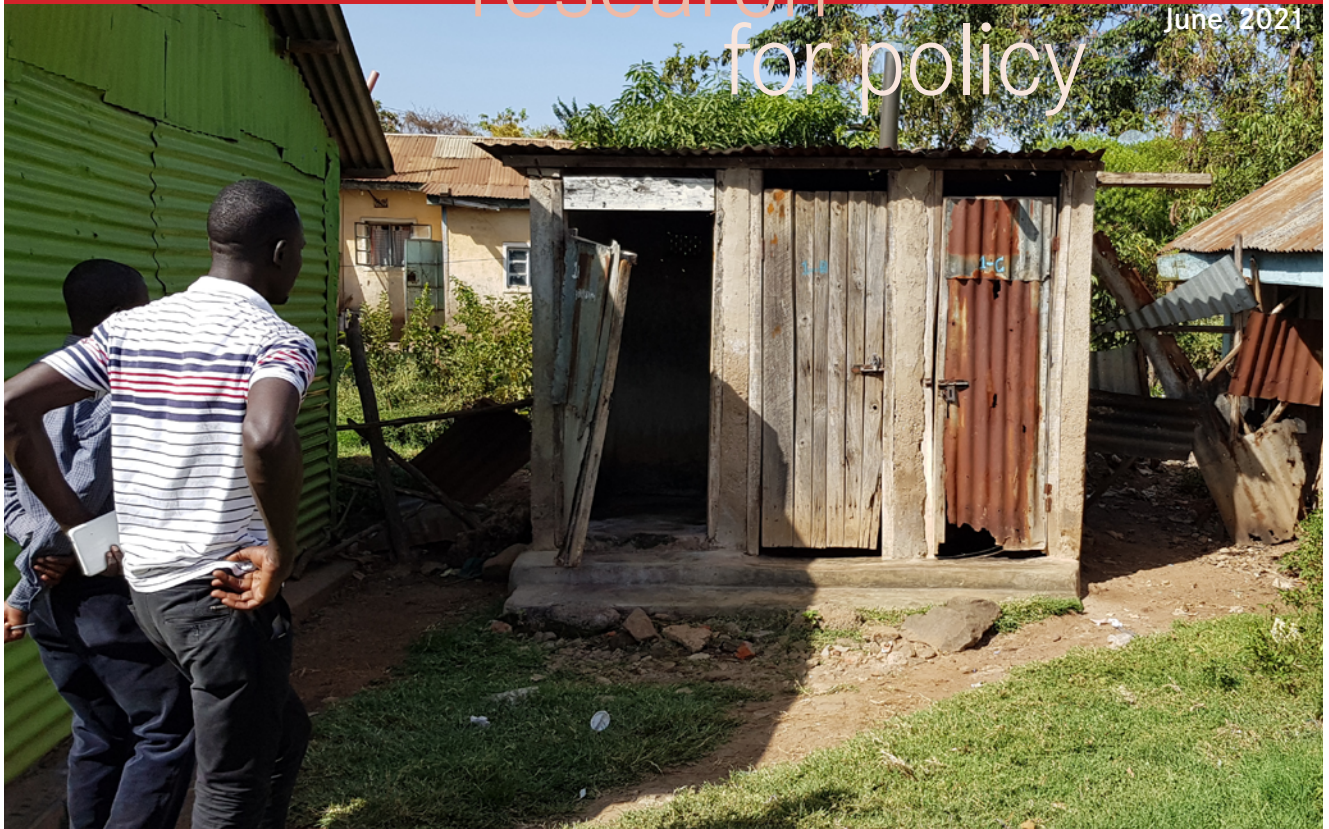
QUISS staff on a site visit to inspect shared sanitation facilities in the low-income area of Manyatta, located in the city of Kisumu, Kenya (Image: Sandec).
