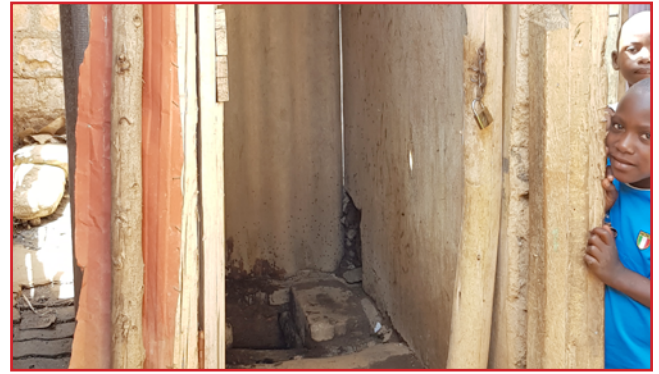
Inspecting shared sanitation facilities in Kisumu, Kenya (Image: Sandec).
