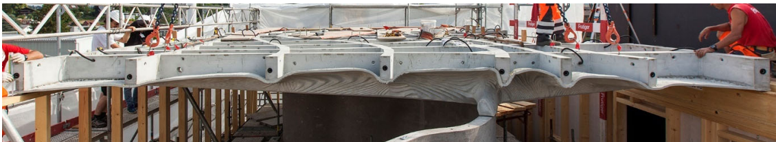
Fig. 2. A section through the Smart Slab shows the variable-height post-tensioned upstand ribs, as well as the ultra-thin interstitial concrete surface.
