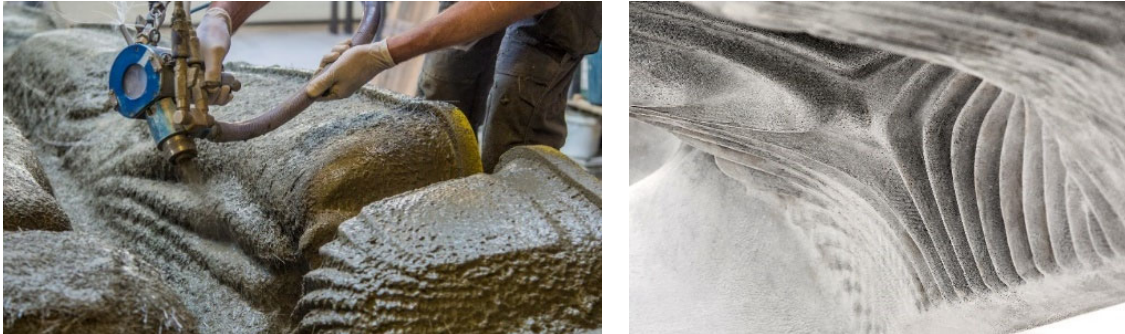
Fig. 3. Concrete spraying (left) and the resulting articulated concrete surface (right).
