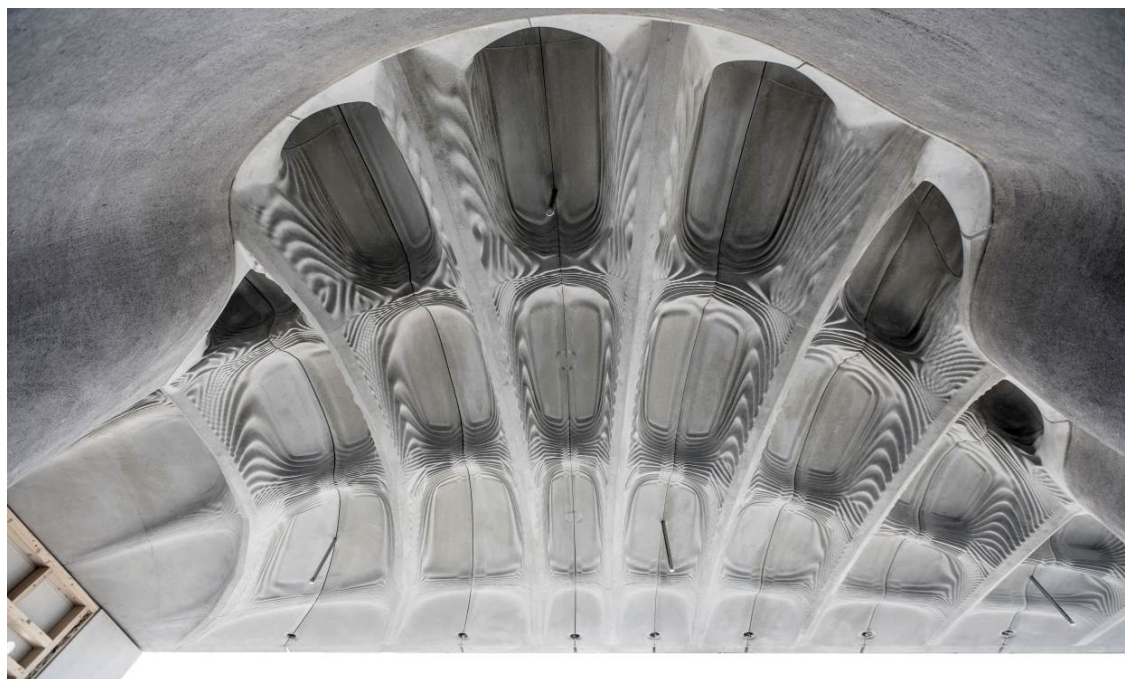
Fig. 1. The Smart Slab – a concrete slab fabricated with 3D-printed formwork.
