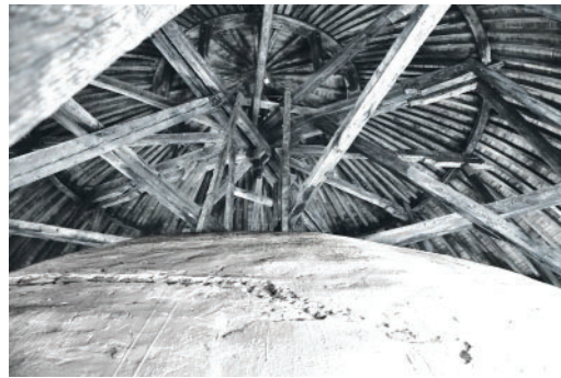
Figure 2. d02. Interior of the attic with the masonry vault and the wooden superstructure (photo: author).
