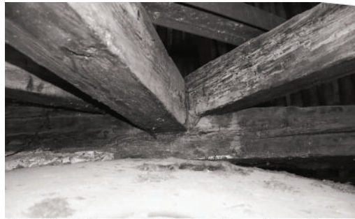
Figure 11. d01: lower collar-beam leaning on the vault's extrados (photo: author).
