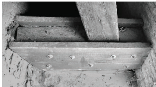
Figure 10. d01, wooden base of a strut placed between the masonry vault and the drum (photo: author).
