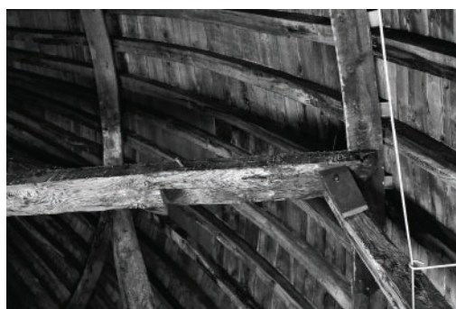
Figure 7. d02: notch visible on the bottom side of a collar-beam (photo: author).
