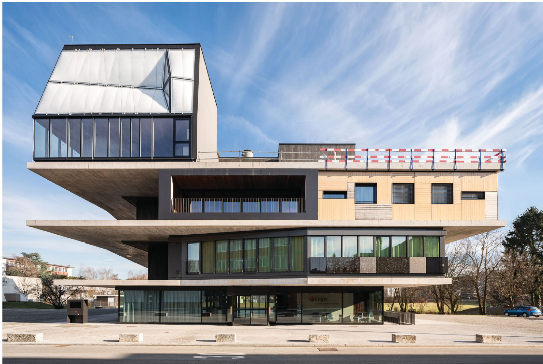
Figure 1. NEST with DFAB HOUSE (upper left).
