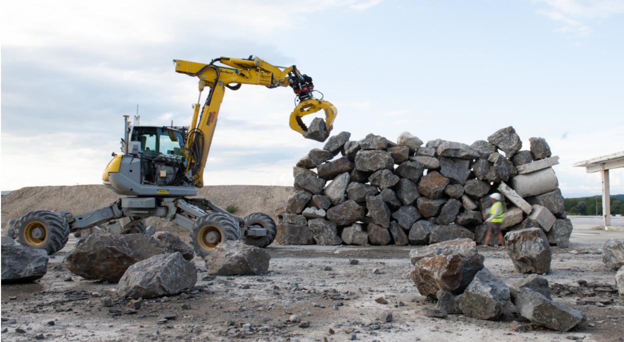
Figure 8.1: The applicability of the proposed grasp approaches in mapping, manipulation, and assembly planning is directly shown in the construction of a large-scale double-faced dry-stone wall with dimensions approx. 10 m x 4 m x 2 m (W x H x D).
