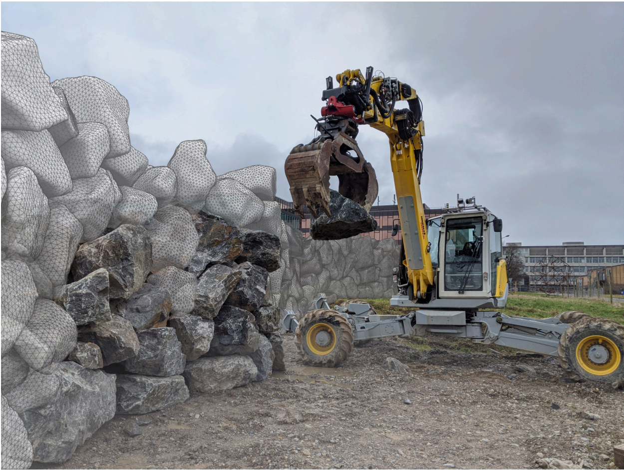
Figure 7.11: In progress wall with overlay of potential extension of structure, generated by allowing the solver to continue with additional digital stone models.
