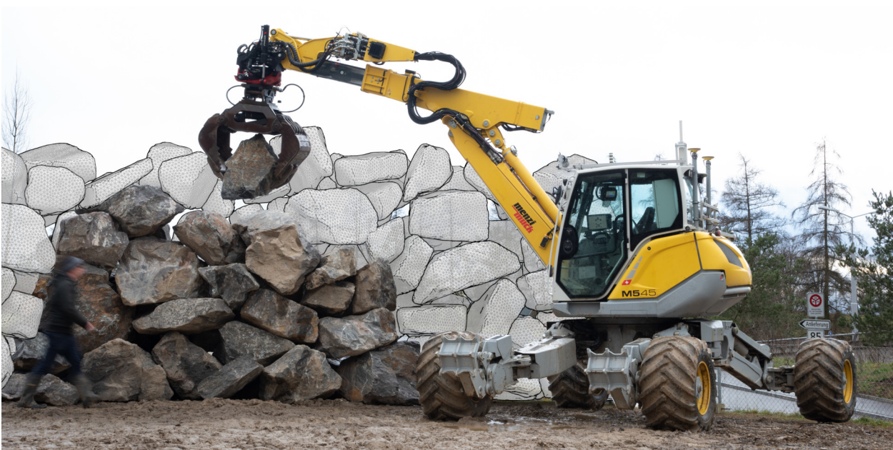
Figure 7.12: Constructed wall with figure (left) for scale and indicated potential extensions.
