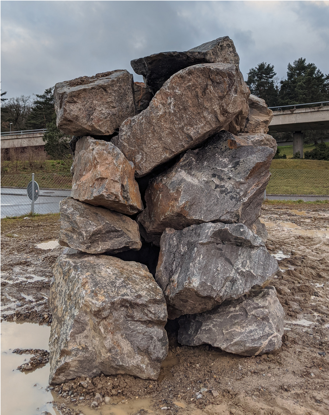
Figure 7.9: Side elevation of constructed wall conveying double-faced structure and near-vertical orientation.
