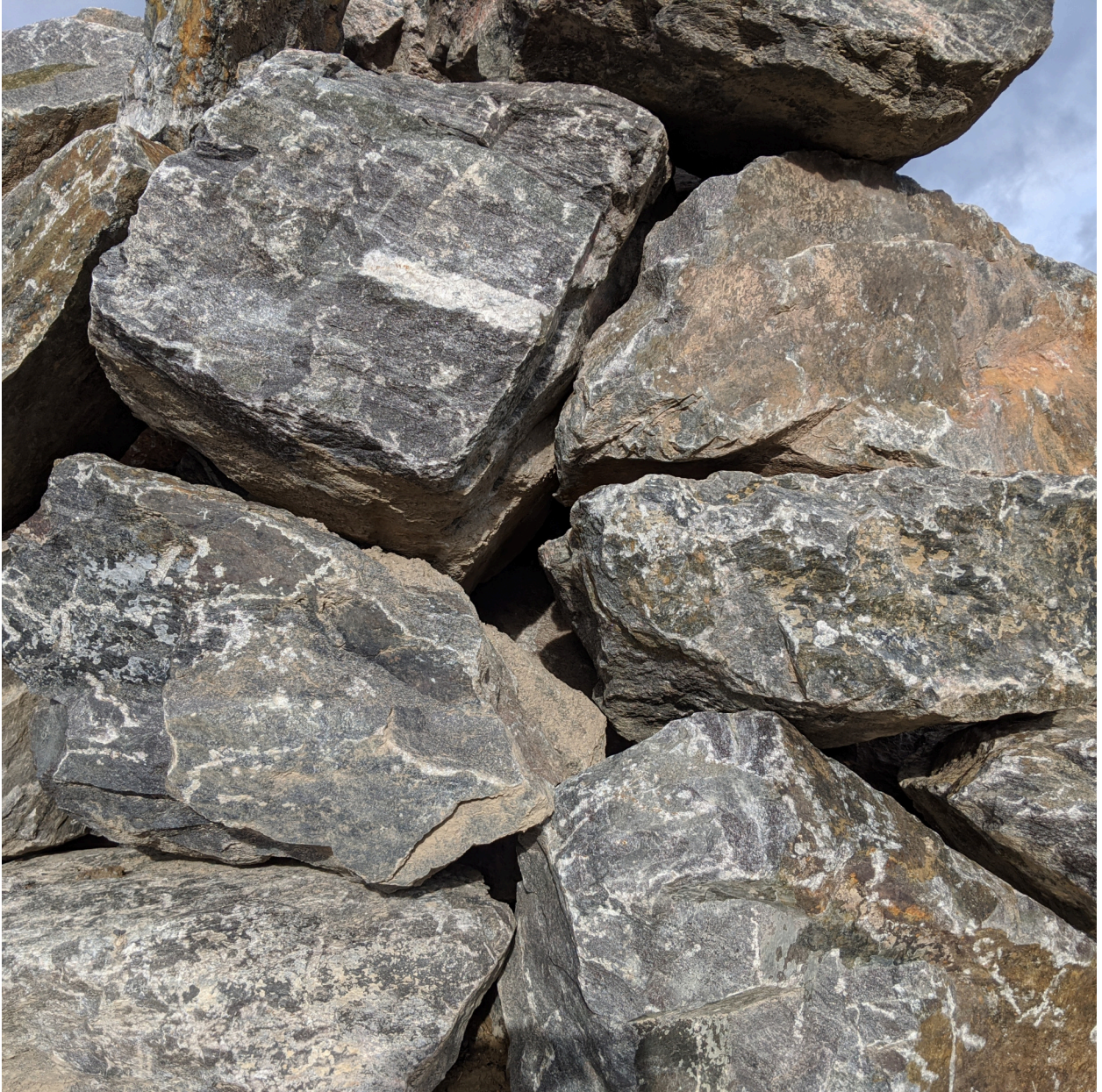
Figure 7.5: Elevation detail of constructed wall. Rotationally invariant shape descriptors allow for a tight fit by initially matching available stone surfaces to corresponding negative geometry of the wall.
