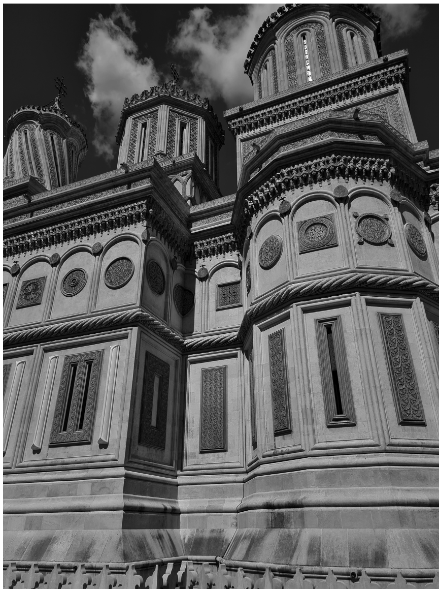
Figure 3.8 Church of Curtea de Argeș, 1515–17: detail of the southern façade.
