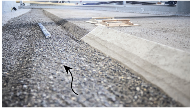
Figure 4.3 Channel after removal of the fixed bank panels to allow lateral erosion of the adjacent floodplain.
