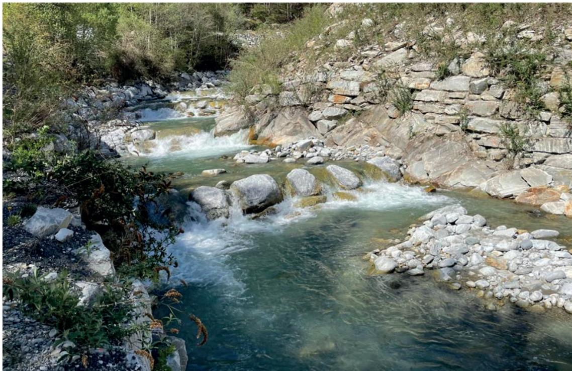
**Figure 3.12** Artificial step-pool sequence in Maira Stream (GR) in 2022; view against flow direction (Photo: C. Tognacca)
