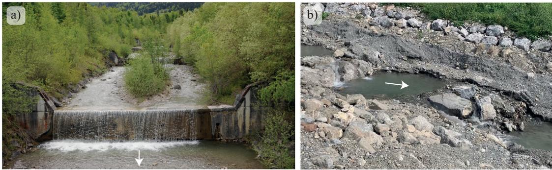
**Figure 1.2** a) Section of concrete check dams in Gürbe Stream, Switzerland,  $S \approx 0.07$  (Photo: SWV 2021); b) Artificial step-pool sequence in Betelriedgraben Stream, Switzerland,  $S = 0.15$ , right after construction in August 2022 at low discharge (Photo: VAW)
