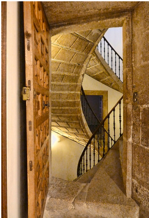
Fig. 1. Picture of a tread in correspondence of a door opening in the spiral staircase of the convent of San Domingo de Bonaval, Santiago de Compostela, Spain, XVII century.
