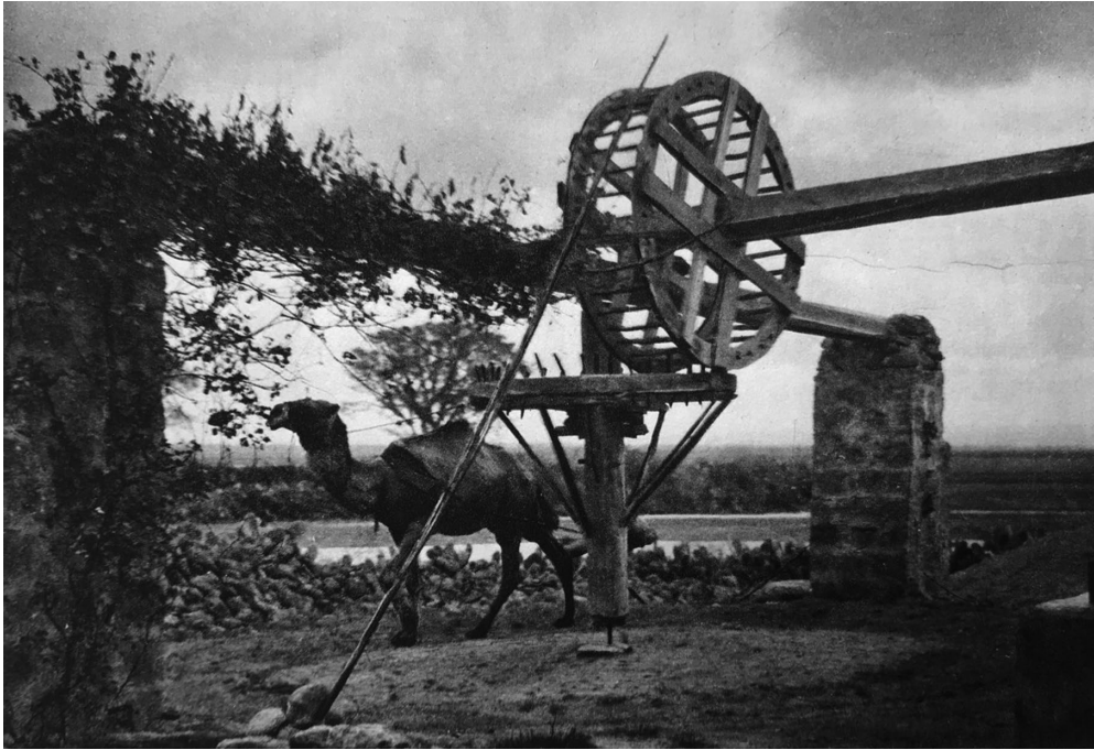
Figure 3. Photograph of Persian wheel water system in Jaffa's citrus plantations. SOURCE: Frank Scholten, La Palestine illustrée , 1929.
