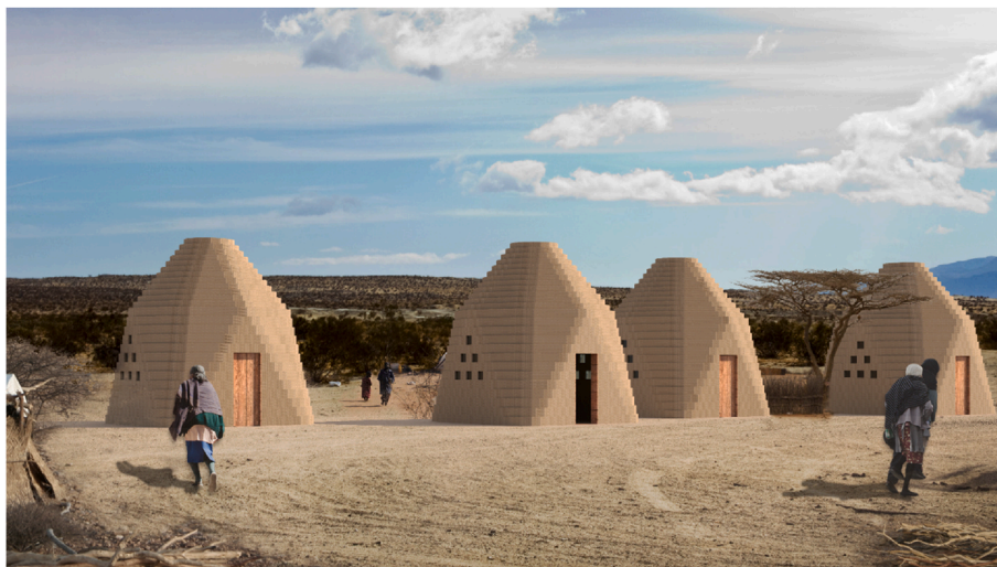
Fig. 13. Conceptual rendering of the 12RA dwelling with triple-course wall zones and double-course roof zones, with small windows. Picture credit to Anastasia Skorik.
