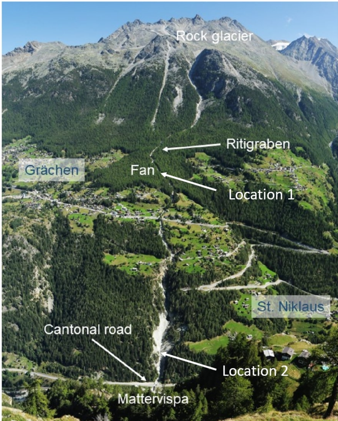
Figure 4.8: Map of the Ritigraben debris flow site. The original map can be found in [140]
