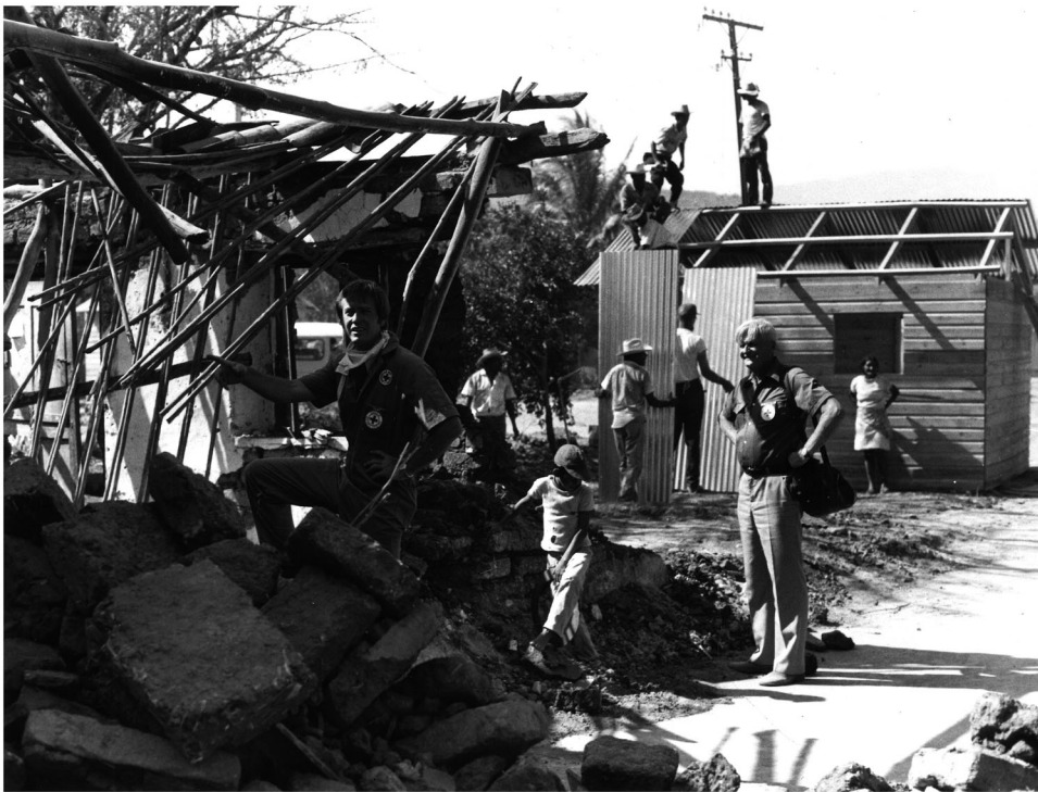
Figure 6. In the foreground, a destroyed house; in the background, a casita in El Progreso, built with materials provided by the Red Cross. The roof is being covered with corrugated metal sheets. Source: Swiss Red Cross Archives. The Swiss Red Cross (SRC) has made six images available for use in this academic article, depicting the intervention in Guatemala following the 1976 earthquake. The SRC understands these images to be free of rights and free of charge. The SRC is not aware of any third-party claims arising from copyright or licenses. It cannot, therefore, be held liable for any claims by third parties. Reuse is not permitted.
