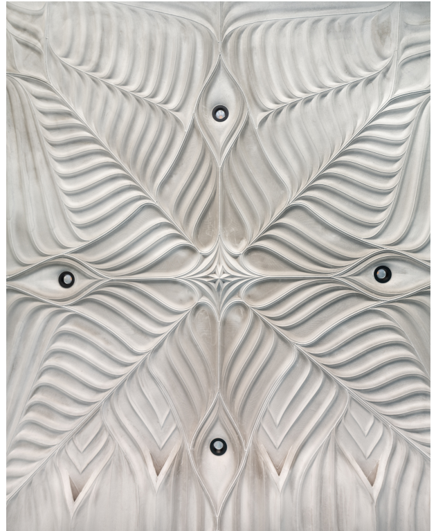
Figure 2: View of the lightweight floor with integrated TABS and ventilation system in office 2, the four air outlets are at the bottom. Photo: Roman Keller.
