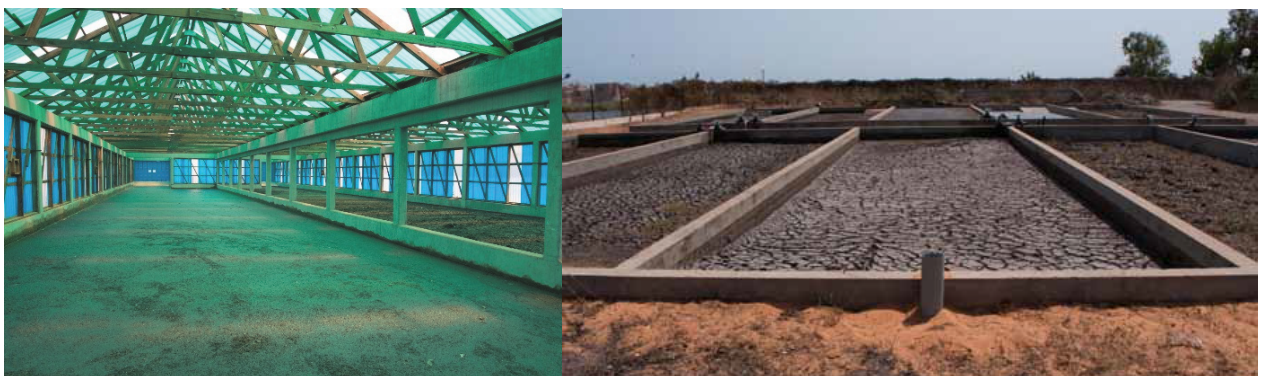
(a) Settling-thickening tanks
