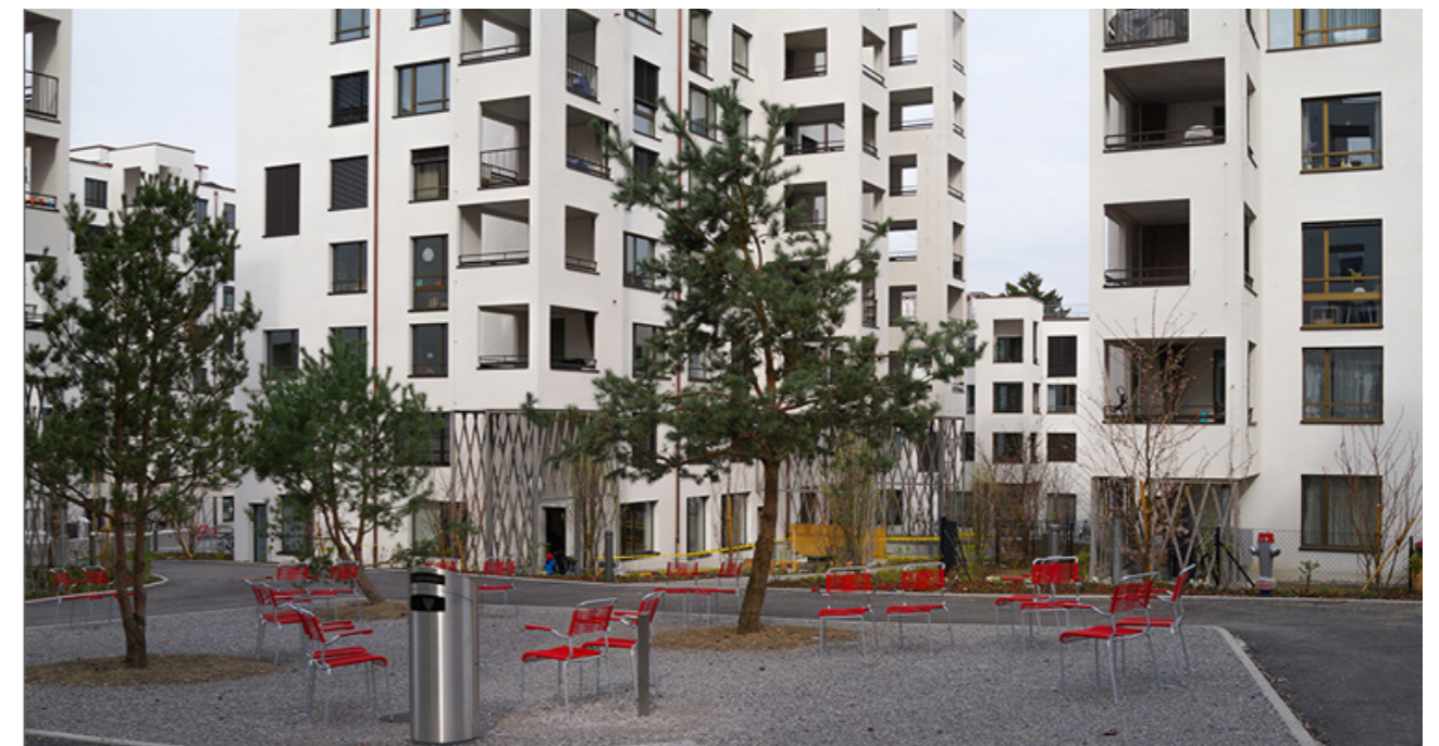
Fig. 4.3.12B: Building project Triemli 1 (Rotach 2023)
