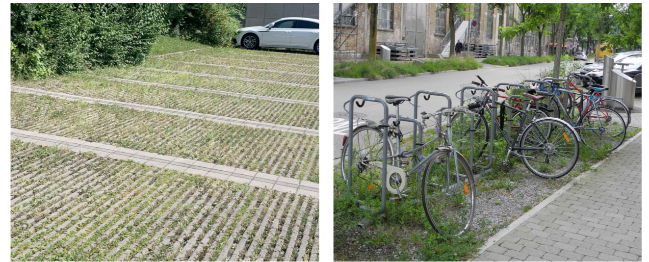
Fig. 4.3.7D: On the left parking spaces with grass liner (Dietlikon) on the right side bicycle parking spaces in a green gravel surface (Zurich) (Tiefbauamt Stadt Zürich 2021).
