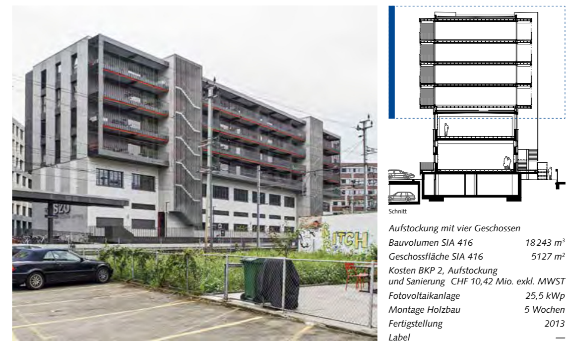
Fig. 4.3.13C: Adding of four storeys out of wood on building (Lignum 2009)
